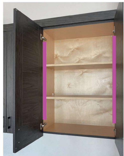
Install fixture between hinges
